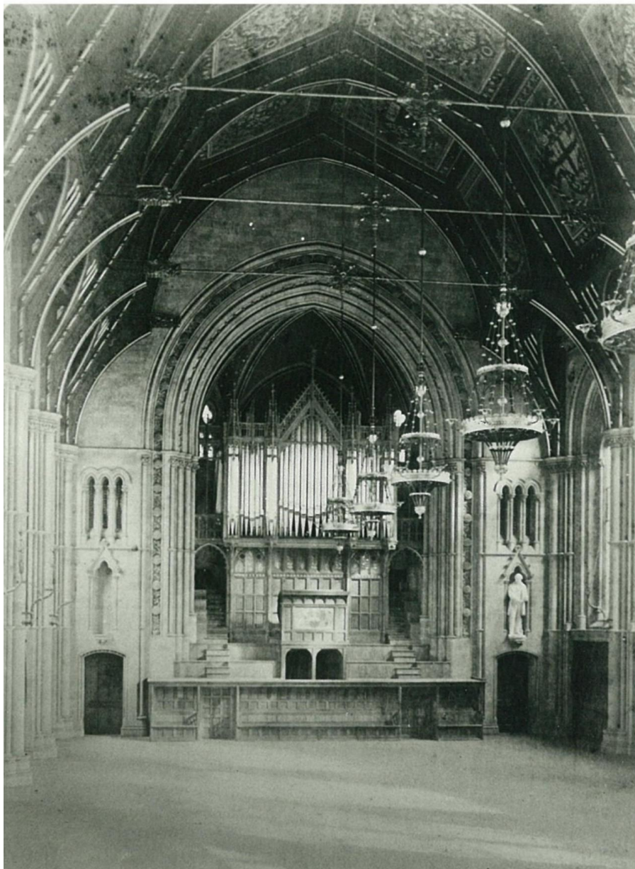
The original appearance of the organ, which will be reconstructed
